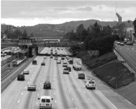
On the Wilson overpass looking west.
