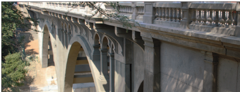
This photo exposes the structural underpinnings of the newly repaired and seismically retrofitted John K. Van de Kamp bridge, which was previously known as the La Loma Bridge.
