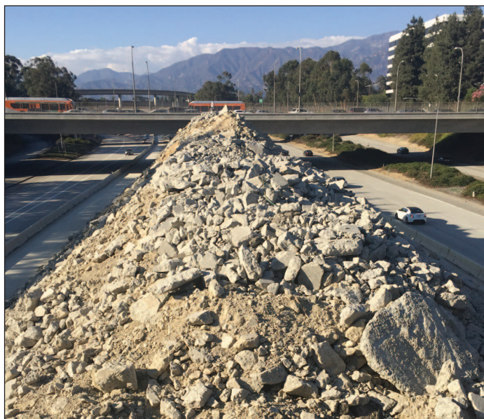
For the past two years Caltrans has piled crushed stone and concrete high — while generating dirt, dust, noise and visual blight — within the Pasadena end of the 710 stub. The batch plant then trucks those materials for use elsewhere to serve as roadbed. (Photo by Chuck Hudson)
