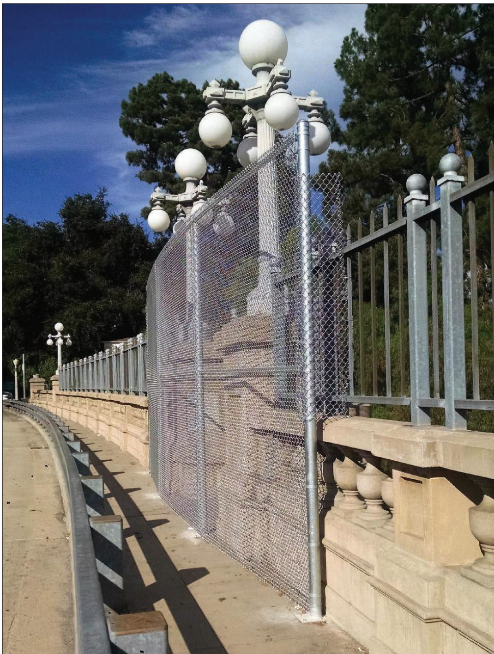
Colorado Street Bridge with barricades
