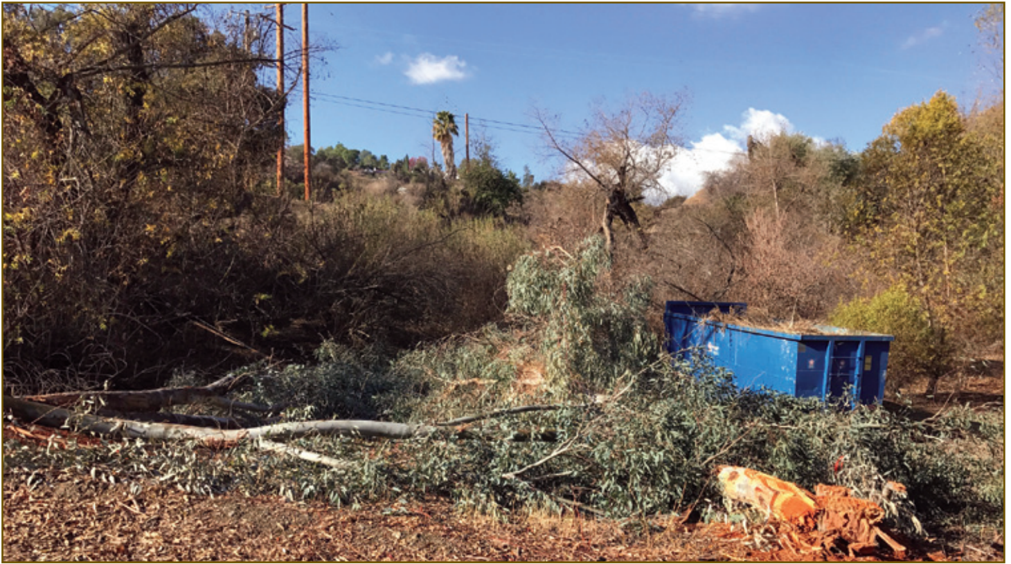
Staging for destruction
