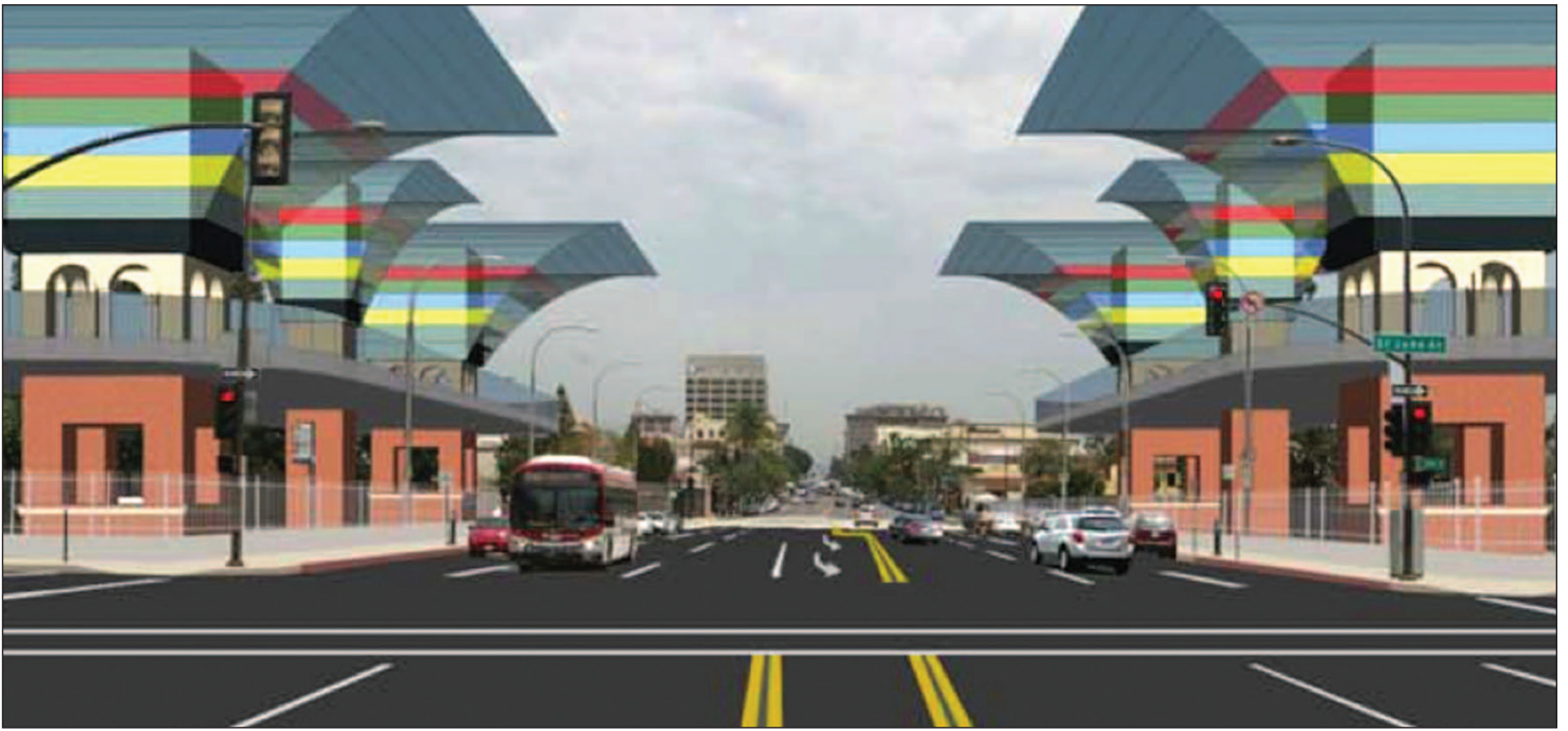
Metro's vision of Colorado Boulevard looking east from Saint John Ave toward Old Pasadena. Six exhaust towers rise from below the bridge to vent the northbound tunnel's exhaust at near street level. (Source: Caltrans and LA Metro's SR-710 Draft Environmental Impact Report / Environmental Impact Statement, Visual Impact Assessment, pg. 204.)
