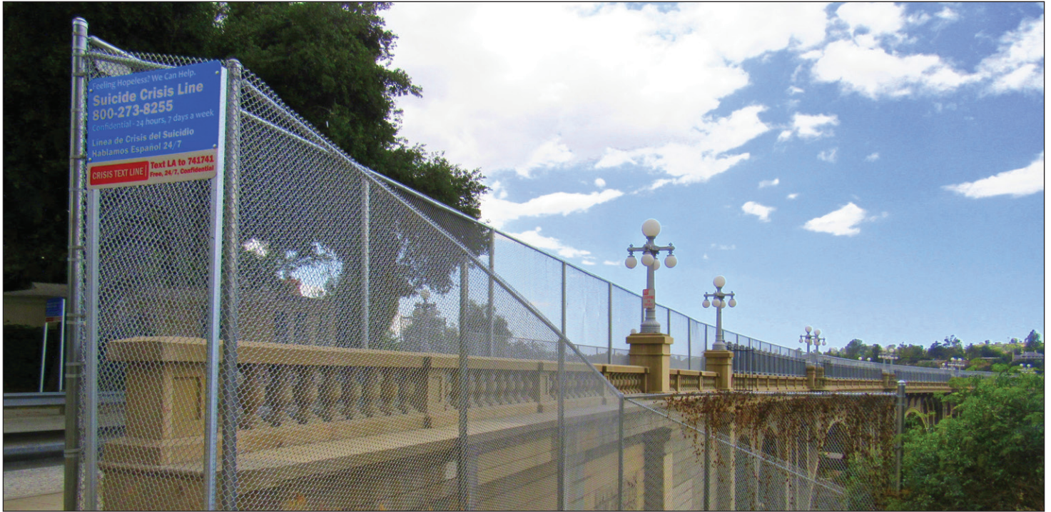
The current temporary fencing on the Colorado Street Bridge (in this photo) will ultimately be replaced by a permanent suicide-deterrent system. Photo by Avram Gold.
