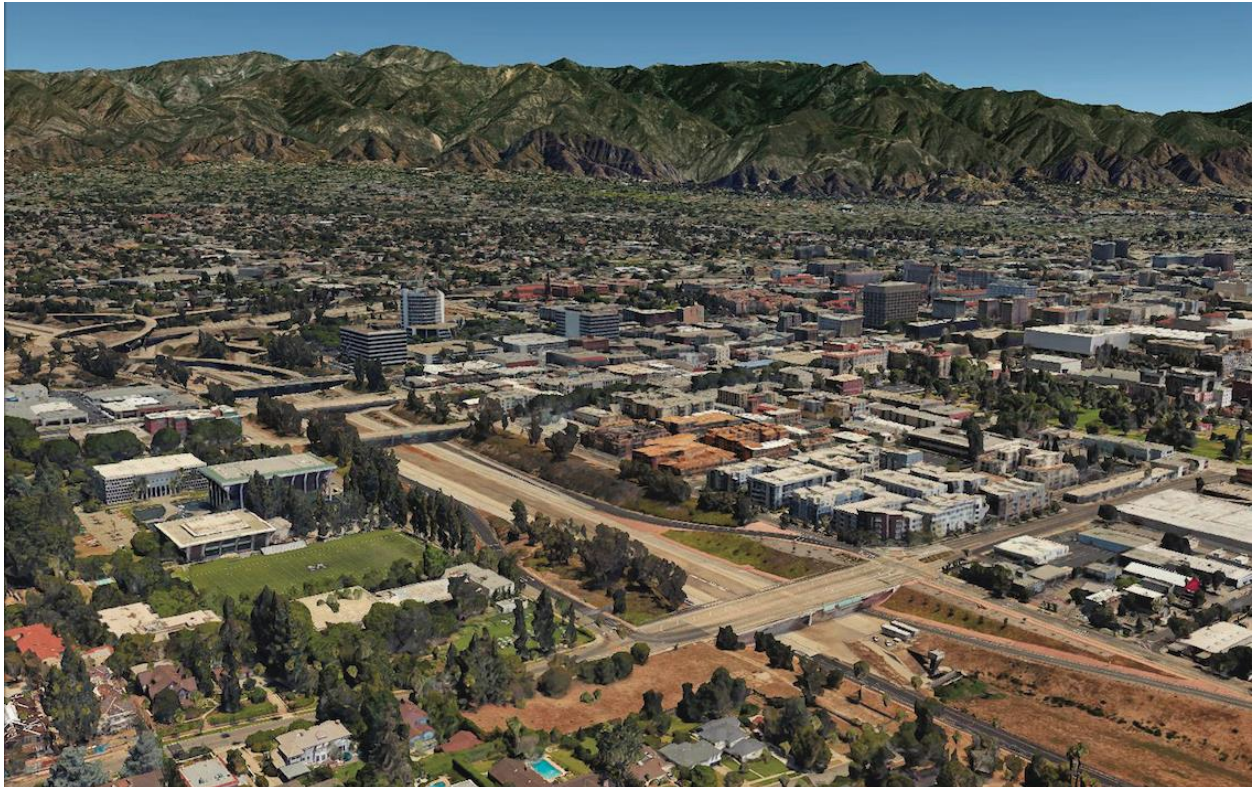
Aerial view of the SR 710 stub.
