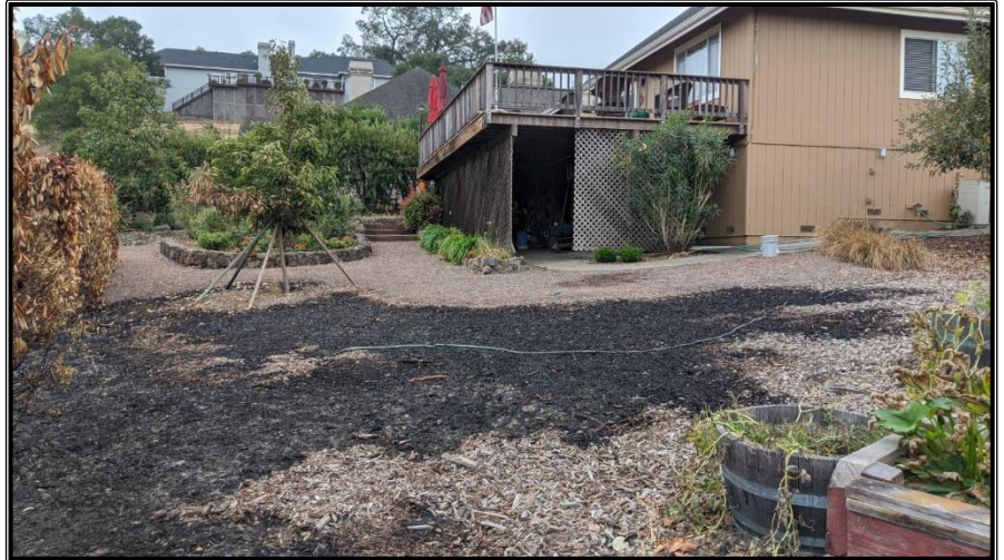
Figure 9: Bark mulch burned up to gravel landscaping adjacent to house during Glass Fire. Note: Homeowner had bark mulch removed and replaced with rock landscaping only two weeks prior to start of Glass Fire.
